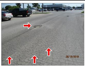
D. Item 1(Picture) Patching and sealing required in the easement
